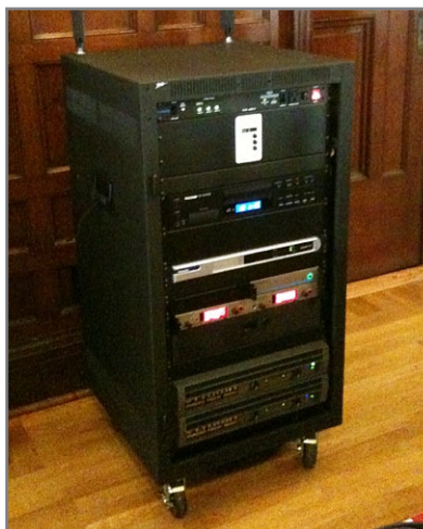
The dining room at Flagler College in Flagler County, Florida, required sound reinforcement that would blend in with the room's design and architecture. Florida Sound built this rolling equipment cart for the dining room.
